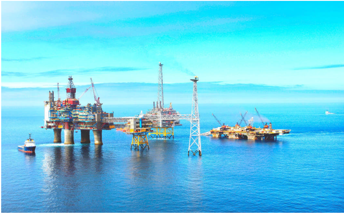
Figure 3: LB200 lays pipe near Sleipner platform summer 2005
